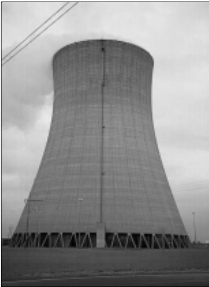
A typical natural draft cooling tower for either a boiling water or pressurized water nuclear power station.
